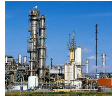
Distributed Control Systems(DCS) Process Control Systems (PCS)
